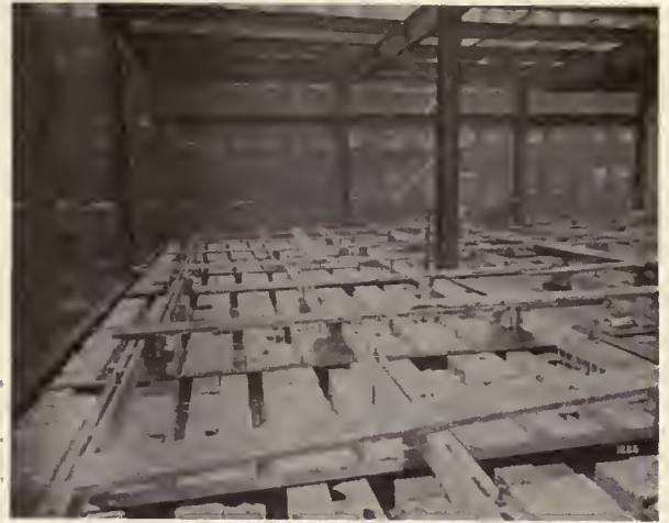
VIEW SHOWING CONSTRUCTION OF FLOOR ARCHES
